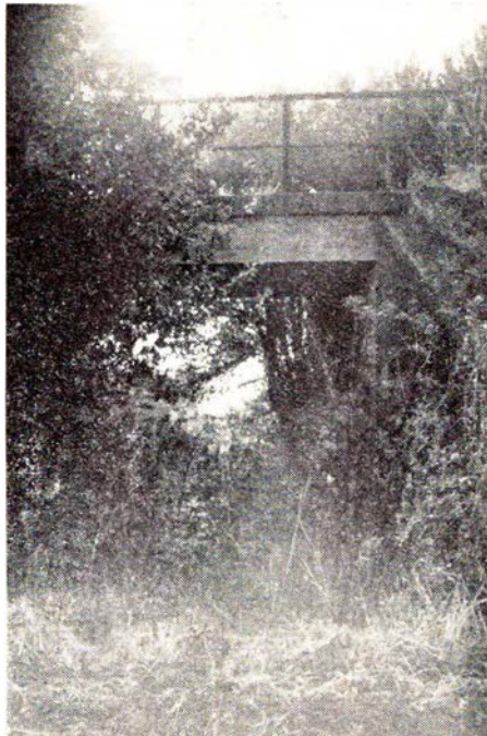
Roebane viadukt under Torrige-banen
